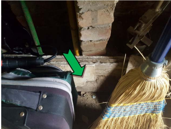
Photo 7. Interior, ground floor, storage area, redundant panels – non asbestos-containing fibre cement sheeting.
