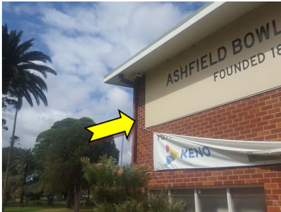
Photo 21. Exterior, throughout, pipework and guttering – suspected lead-containing red upper paint system.
