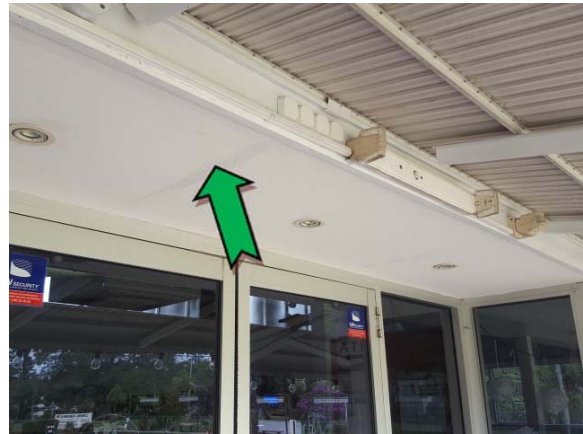
Photo 4. Exterior, main entrance, awning, throughout – non asbestos-containing fibre cement sheeting.
