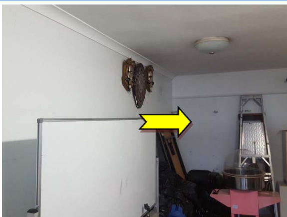
Photo 23. Interior, locker room, throughout, walls – suspected lead-containing blue upper paint system.
